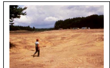
Dry dredging of Dunn's Pond in Gardner complete, with removal to “hard” bottom
