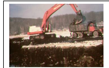
Dry dredging of Dunn's Pond in Gardner with conventional excavation equipment
