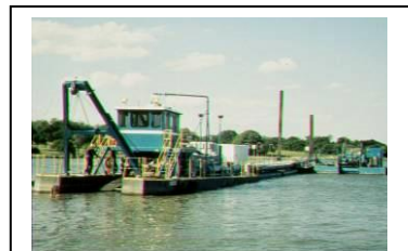
Hydraulic dredging: large cutterhead barge
